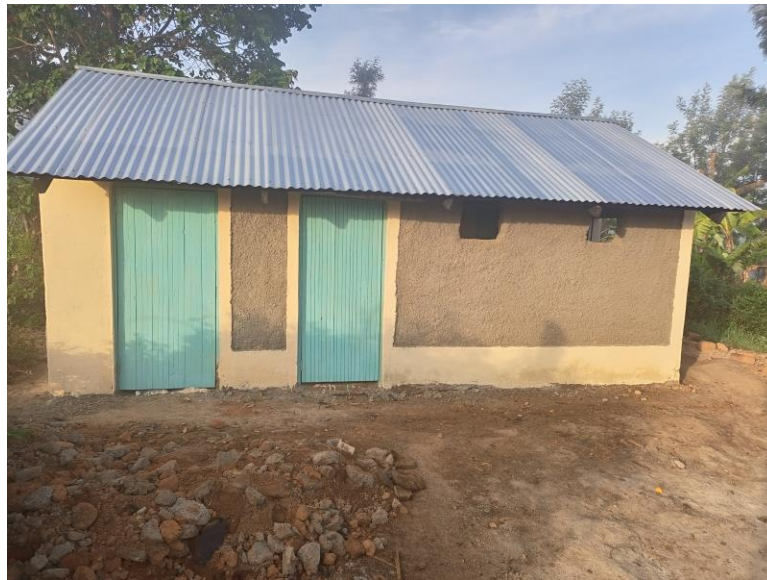
New toilet block at Evaland Academy
