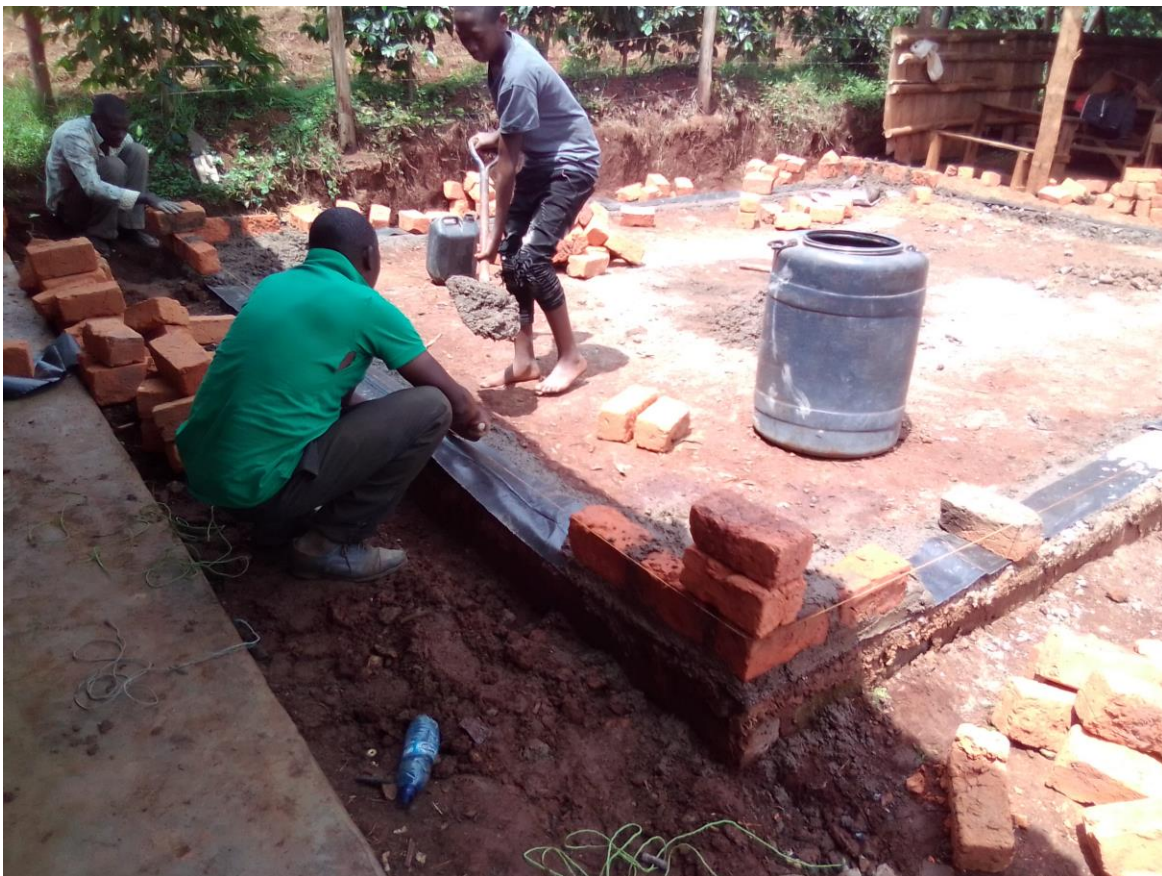
New classroom construction at Surgeon Academy
