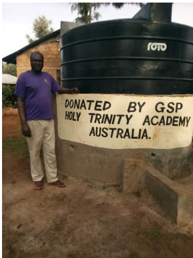
Water tank at Evaland Hekima Academy
